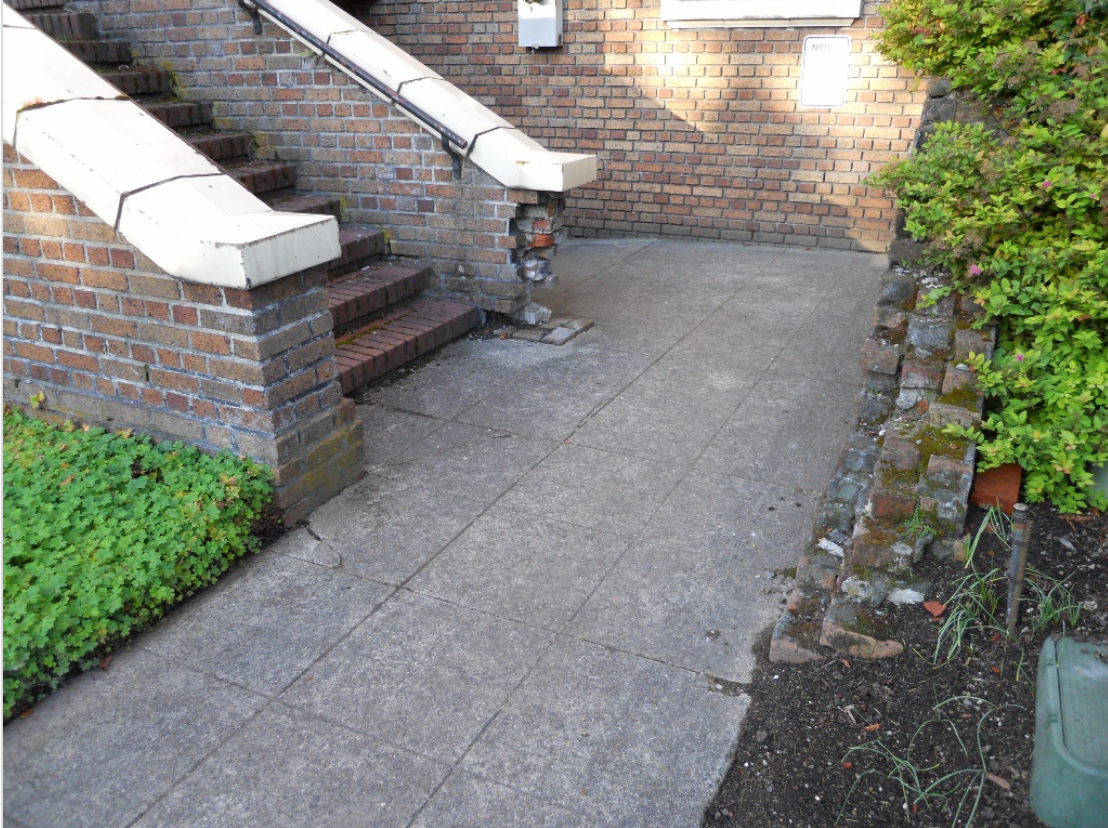
Photo 1: Damaged banister
