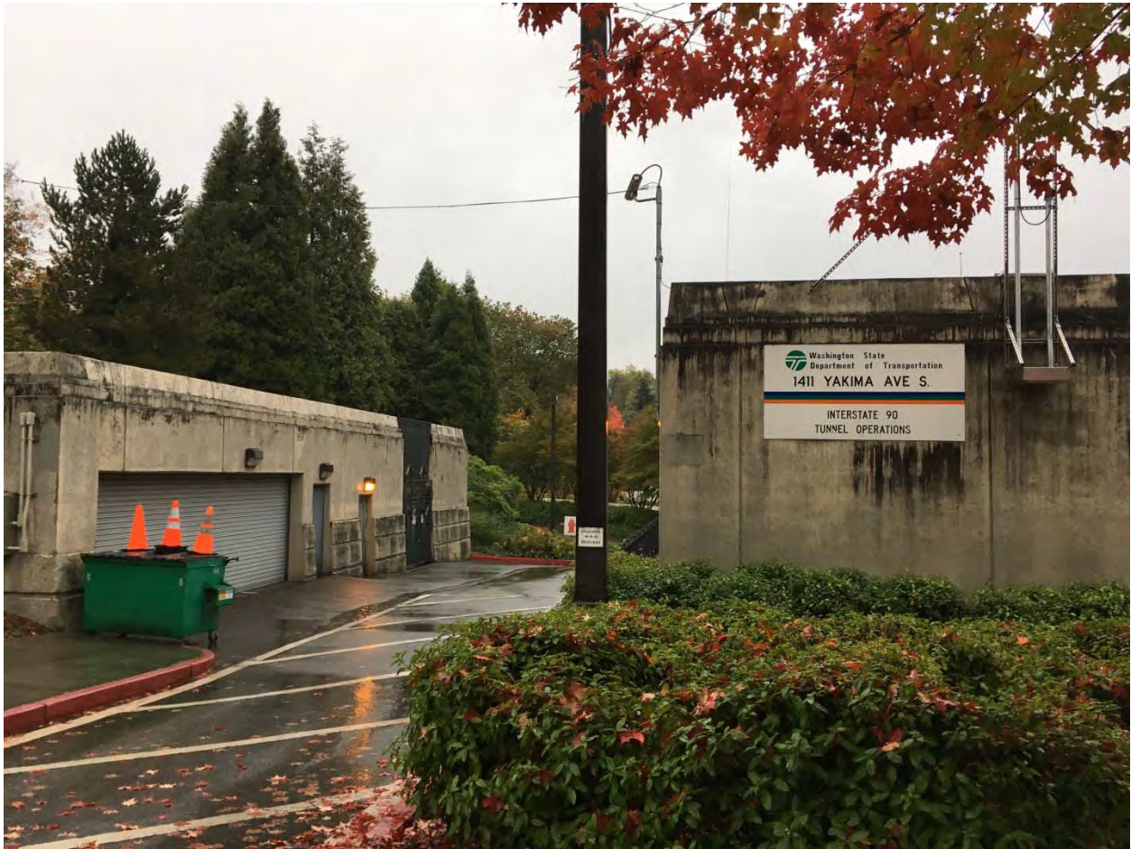
WDOT Interstate 90 Tunnel Operations Facility Located at 1411 Yakima Avenue South (Southwest of the Subject Property)
