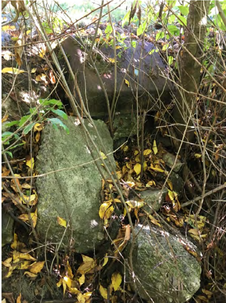
Rubble Fill and Debris on Southwest Portion of Subject Property West of and Below Retaining Wall
