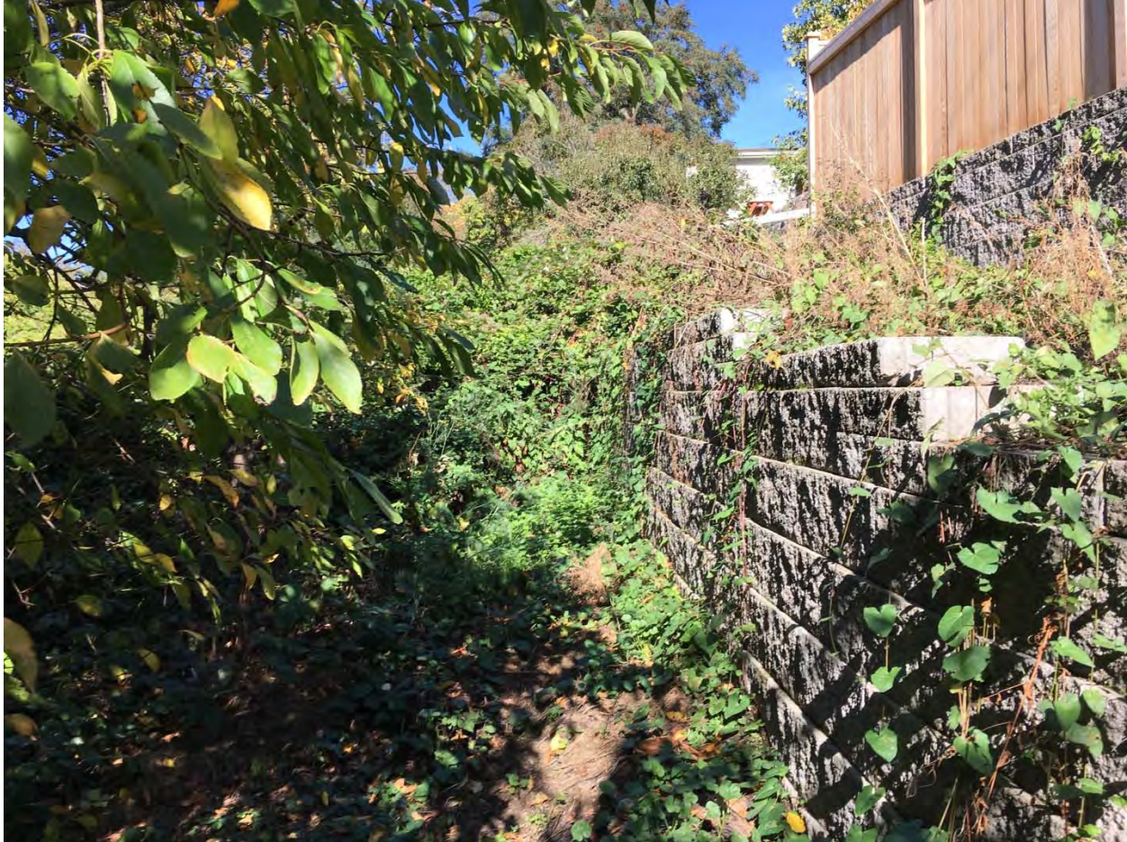
Southeast Corner of Subject Property, Viewing North. Retaining Wall (Front Right) and Rubble Fill Soils (Front Left) Encroach on Subject Property (Assuming the Fence Corresponds to the Approximate Property Line)
