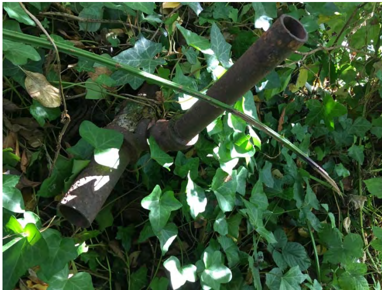
Discarded Sewer Plumbing Associated with Southwest Rubble Fill, Viewing South
