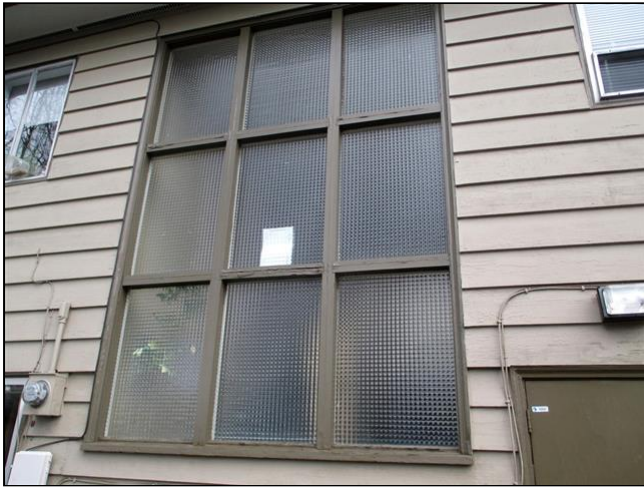
Wood trim is decayed on this window
