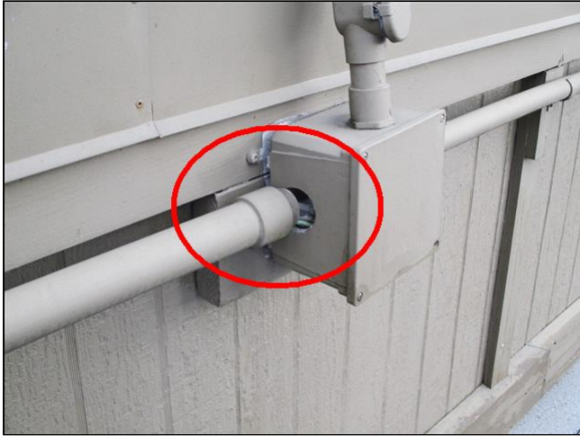
Conduit is disconnected from the junction box
