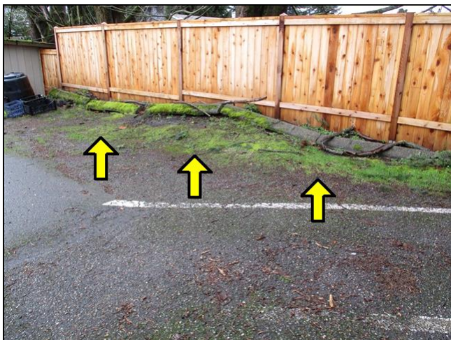
Asphalt parking area is damaged
