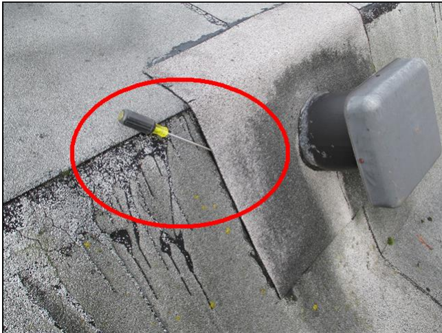
Seams in the roofing materials are not sealed properly
