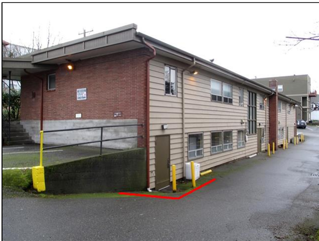
Install an asphalt berm to direct water away from the door
