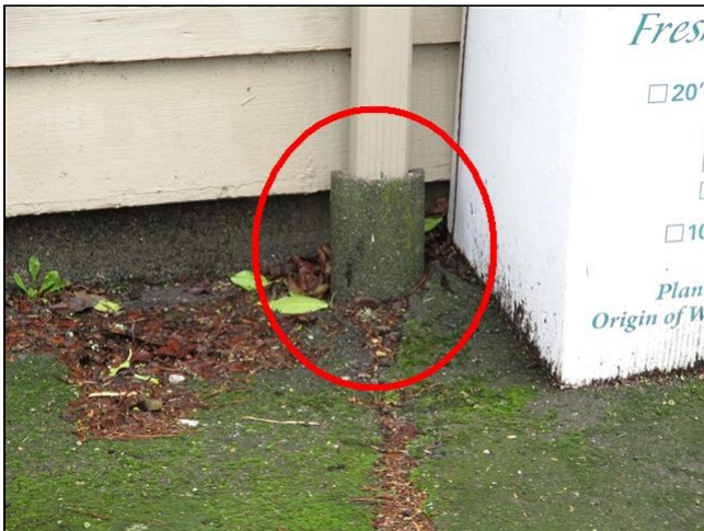
Old concrete drain system
