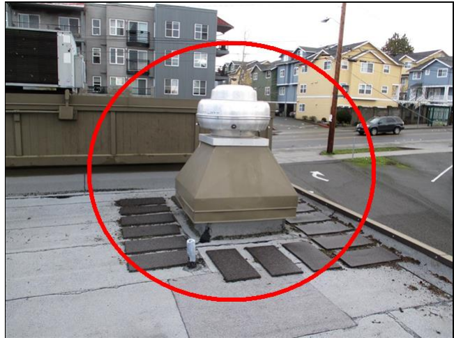
Roof mounted section of the kitchen exhaust fan
