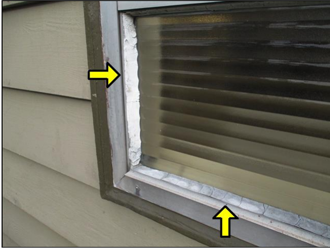
The old windows are in poor condition
