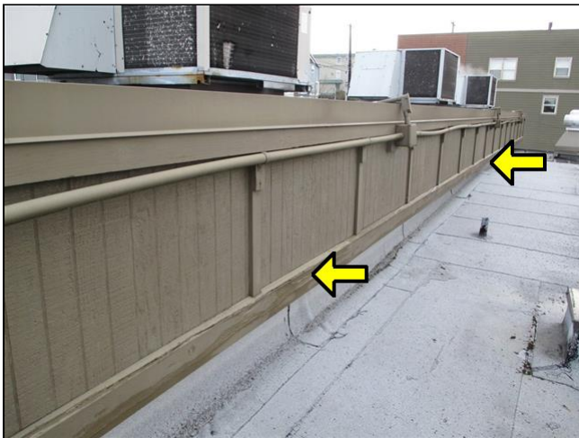
Decayed trim boards
