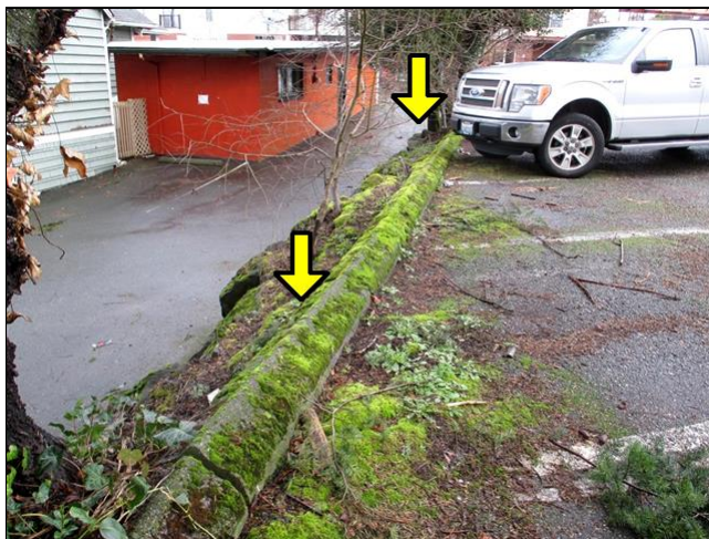
Install a guardrail or larger curb
