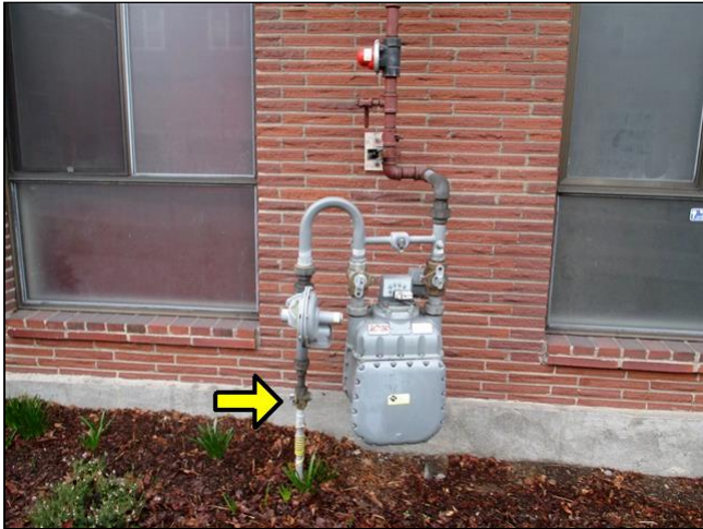
Main gas shutoff valve
