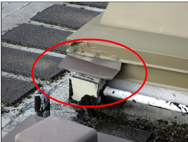
Incorrect flashing installation
