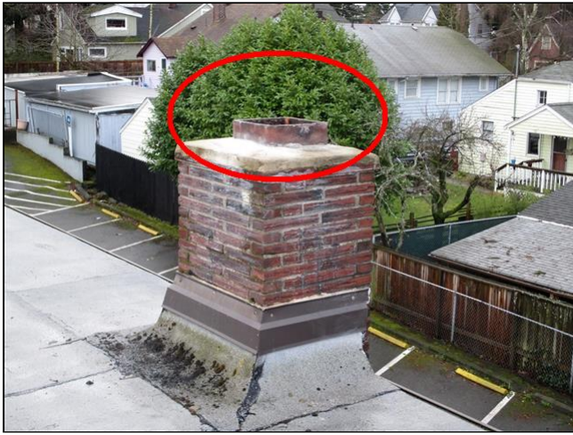
Install a weather cap on the chimney
