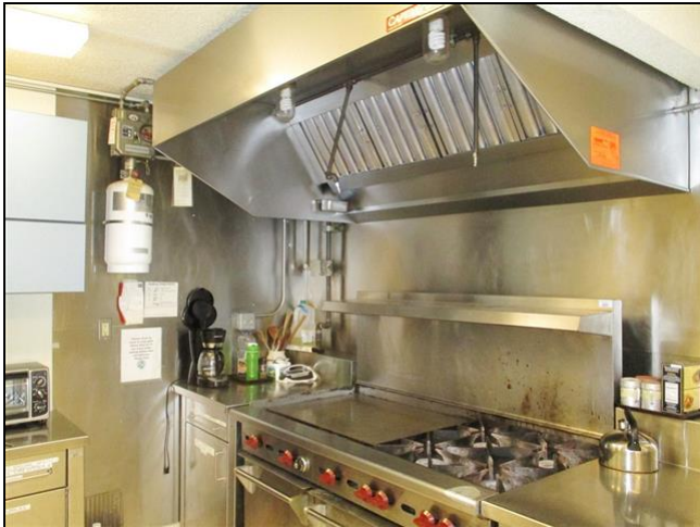
Kitchen exhaust hood in acceptable condition
