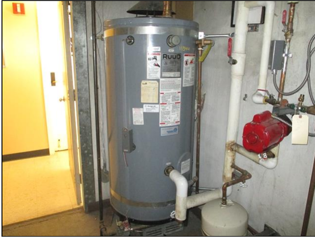
Replace the old water heater
