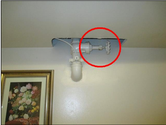
Main water shutoff valve
