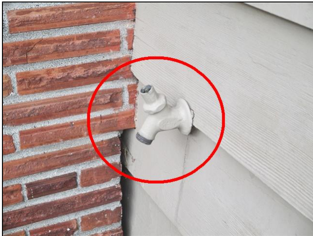
Install an anti-siphon valve
