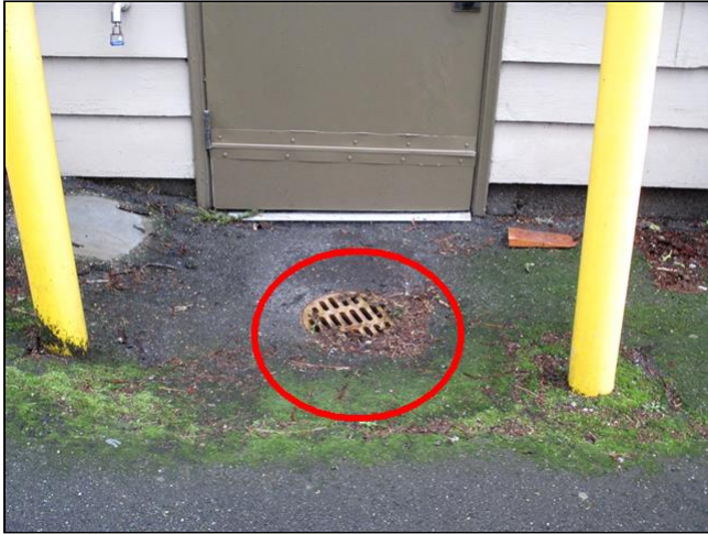
Flush out the storm drain
