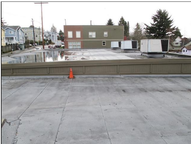
View of the roof
