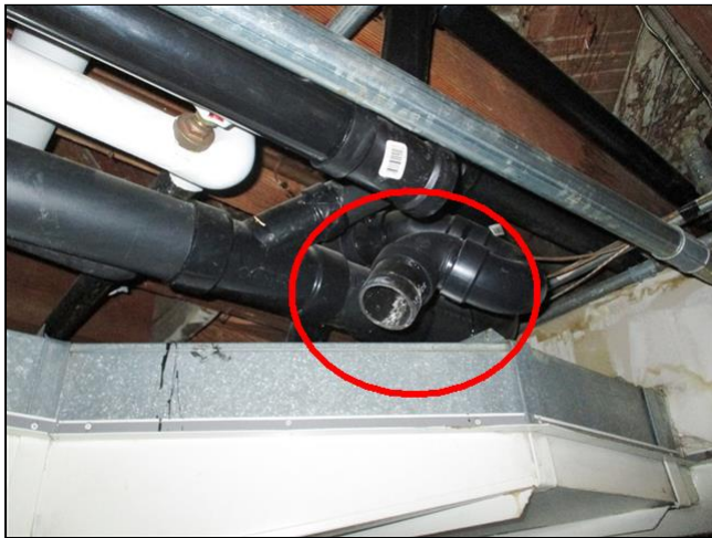
No cap on the end of the drain pipe
