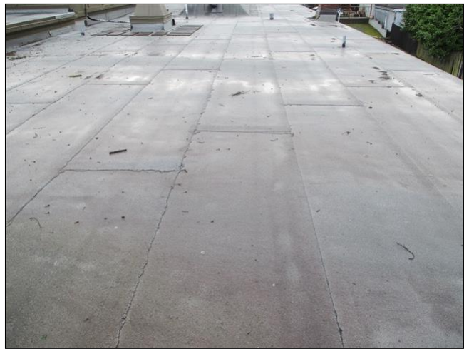
View of the roof
