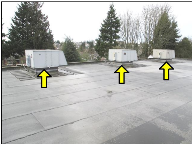
Three heat pumps on the roof
