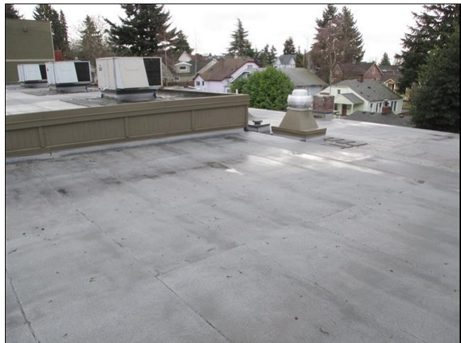
View of the roof
