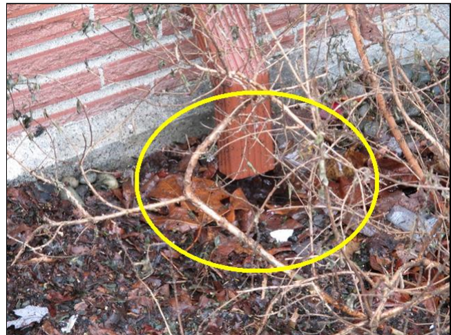
The downspouts discharge at the foundation
