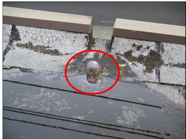
Drains are installed too high
