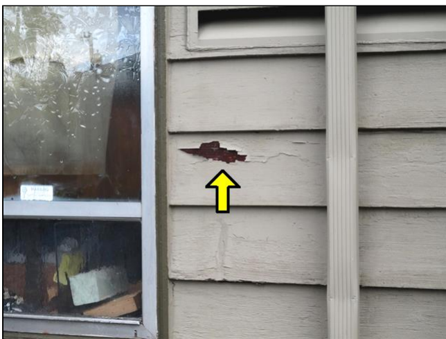
Paint is peeling on the siding
