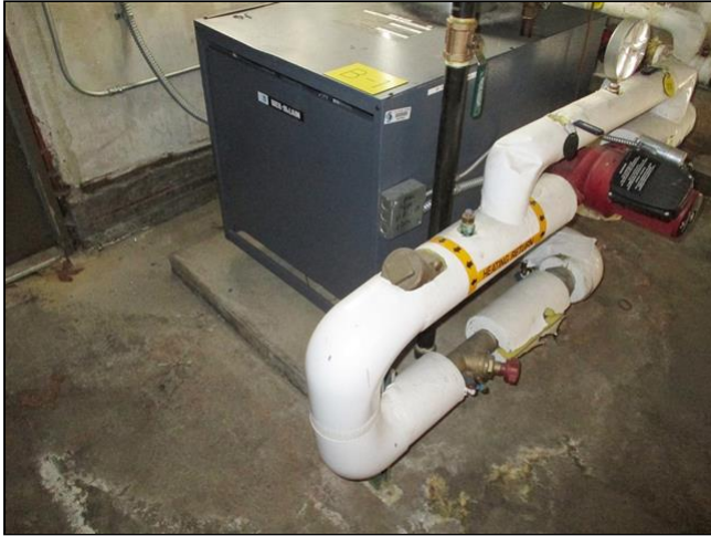
5 year old boiler
