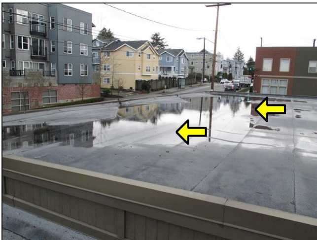
Water is ponding on the roof
