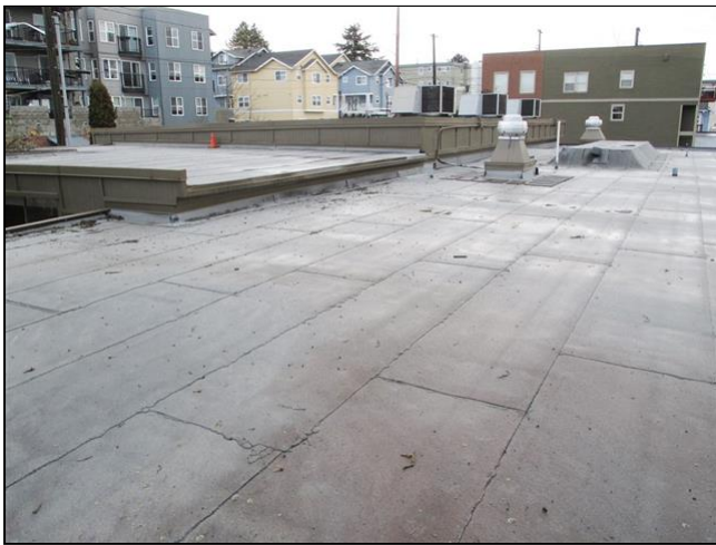
View of the roof
