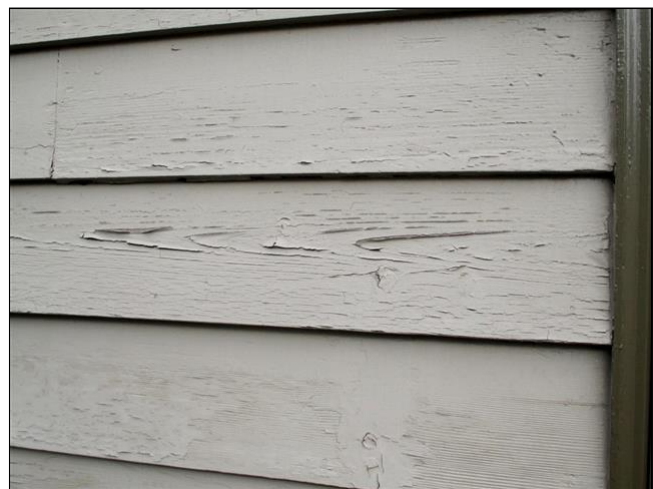
Paint is peeling on the wood siding
