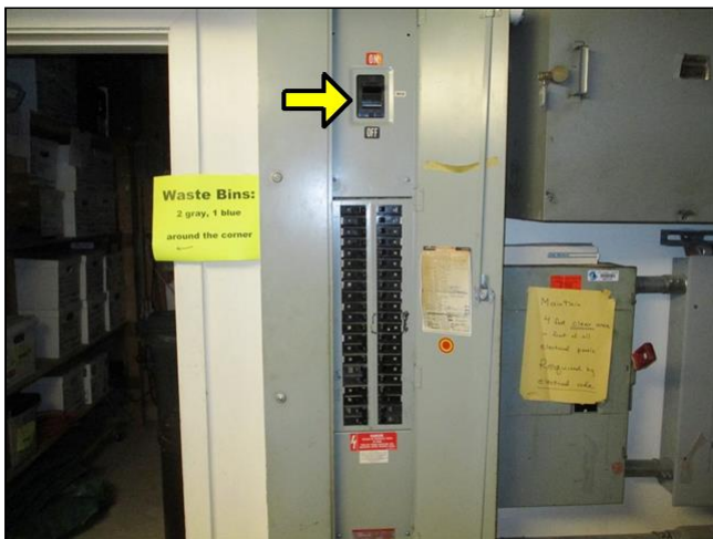
Main electrical disconnect breaker
