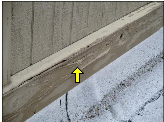
Decayed trim boards
