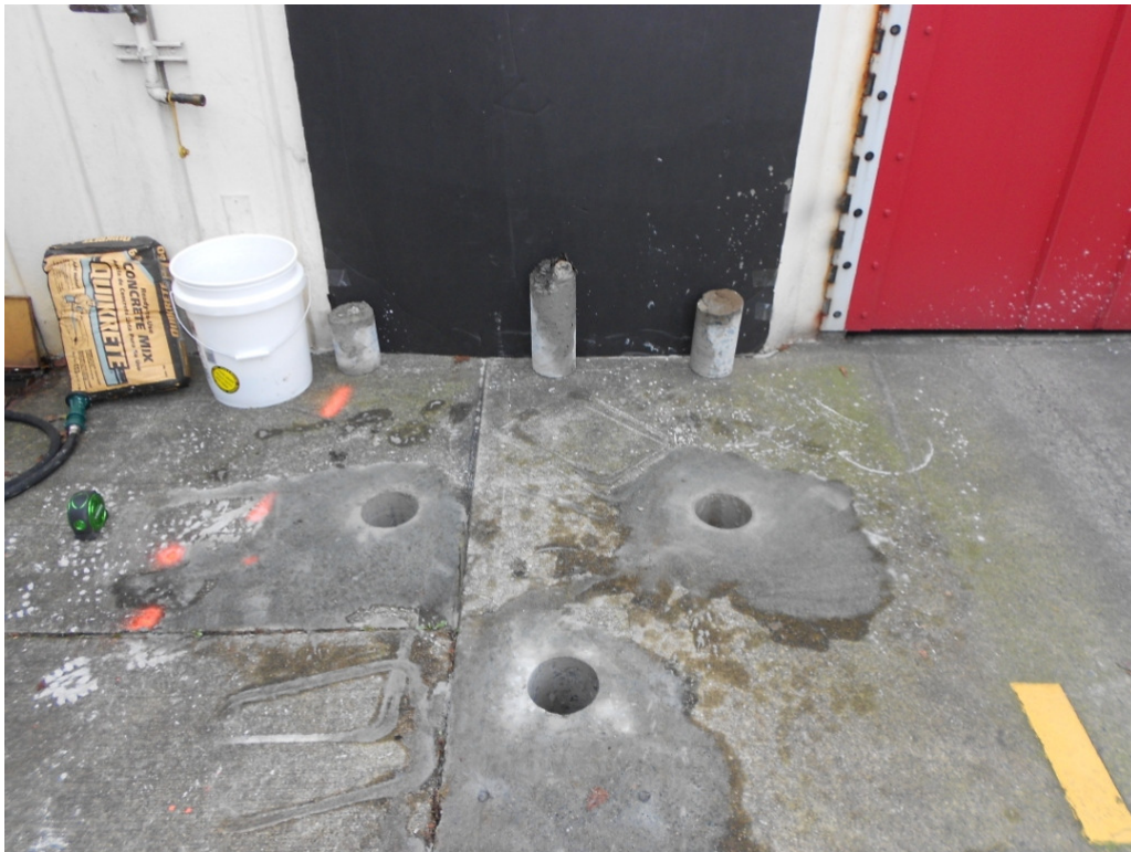
2. Looking west at the borehole locations after concrete coring and prior to hand augering. The boreholes were designated B-1, B-2, and B-3 from left to right, respectively. The concrete cores for each borehole are lined along the Fire Station building adjacent to their respective borehole.
