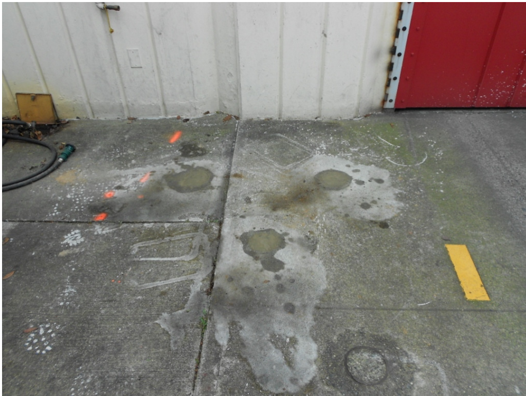
3. Looking west at the borehole after hand augering and the borehole have been sealed with fresh concrete.
