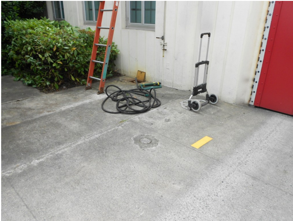
1. Looking southwest at the location of the former UST and fuel dispenser prior to field activities.
