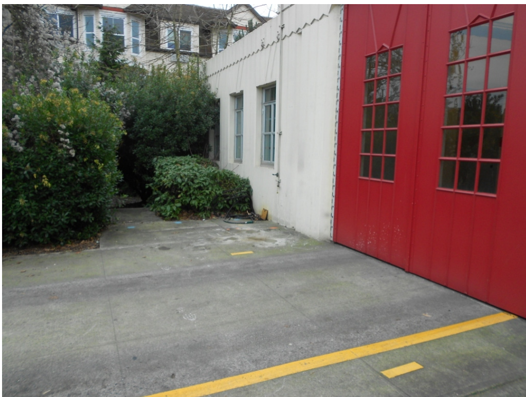
4. Looking southwest at the location of the boreholes after all field activities.
