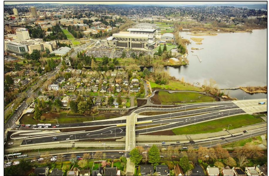
Aerial photo of the SR 520 westbound off-ramps to the Montlake area, looking north. Photo taken: 2017.
