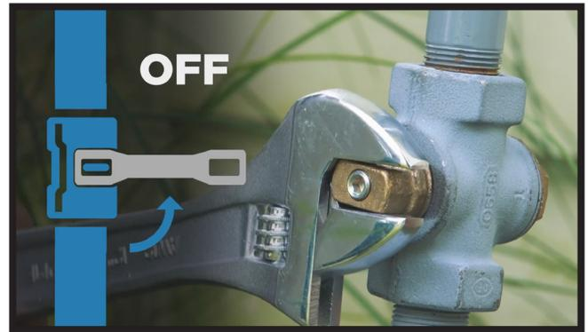
Locate the meter shut-off valve. It's usually the first fitting on the gas supply pipe coming out of the ground near your meter. Use a long-handled wrench to give the valve one-quarter turn in either direction so that the lever is crosswise to the pipe. Once the gas is off, leave it off. Contact your gas company to inspect the system, check the relight appliances.
