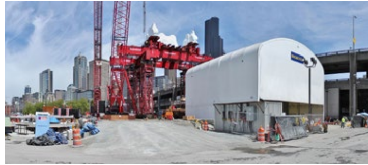
Bertha tunneling machine repair gantry
