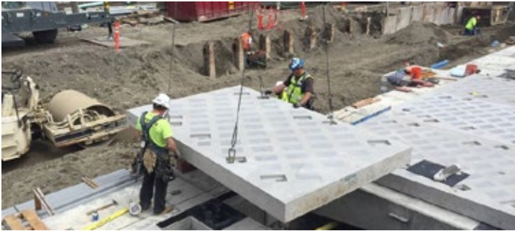
Concrete panels are lowered into place on top of the Zee panels for the seawall
