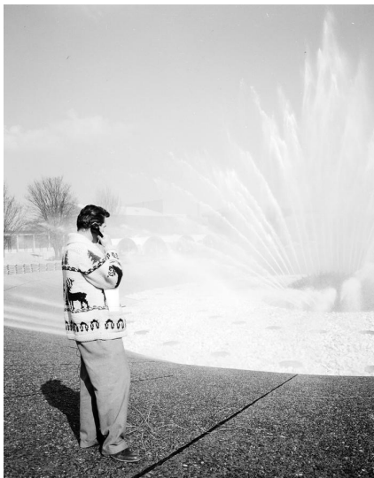
International Fountain, adjusting nozzles, March 12, 1962. Image 195611 , Series 8200-13, SMA.
