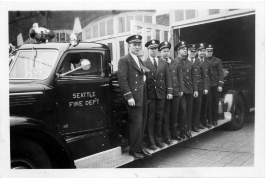
Seattle Fire Department Ladder 3 B shift, 1938 (estimated). Item 195490 , Series 9995-01, SMA.
