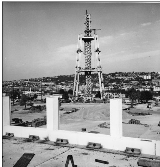
Space Needle construction, 1961 Item 77335, Seattle Municipal Archives
