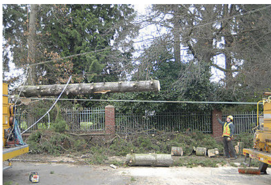
City Light Crew Repairing Wind Storm Damaged Lines from Fallen Tree. E. Madison St. and 37th Ave. E., December 17, 2006. Item 152772
