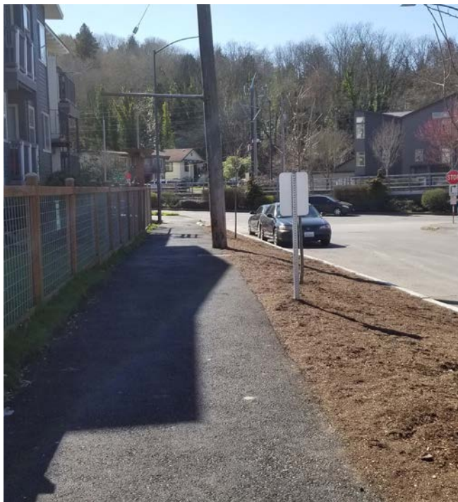
Cost-effective asphalt walkway on S Byron St
