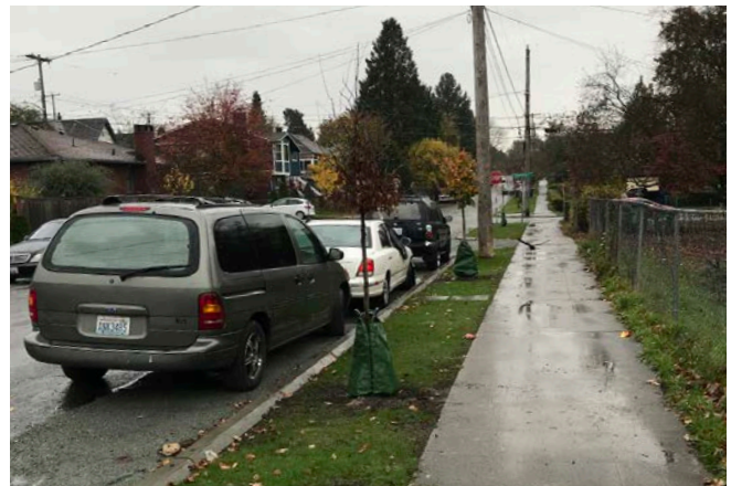
Delineated, at-grade concrete walkways
