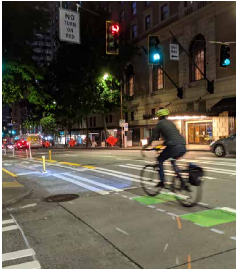
Protected bike lane through the intersection
