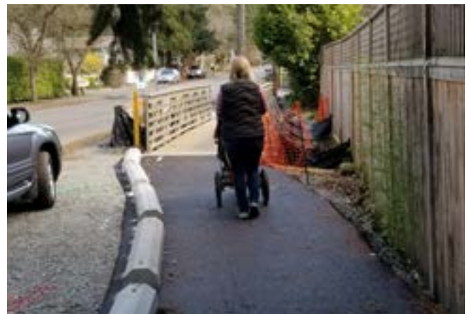
Delineated, at-grade asphalt walkways
