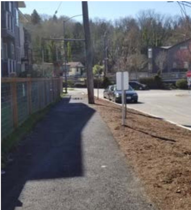
Cost-effective asphalt walkway on S Byron St
