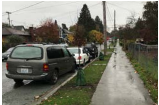
Delineated, at-grade concrete walkways
