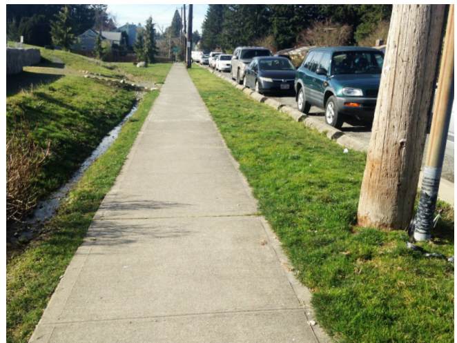
Delineated, at-grade asphalt or concrete walkways
