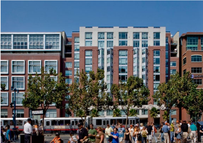
Building modulation breaks up the mass of a building's frontage. When done well, it creates visual interest and can reflect the program inside the building to passersby. (GGLO)
