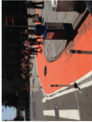
Photo Above: Example of interim curb extension - paint and plastic bollards; Photo Below: Existing curbside on Leary Ave
