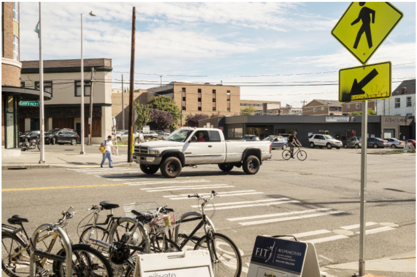
The intersection of Leary Avenue, 20th Avenue, and Vernon Place has five legs approaching at unusual angles.
