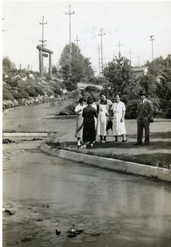
Lily Pond with the Rockery Wall Showcase and Entry Gate in background Source: KGF Photo #1983, dated 1935
