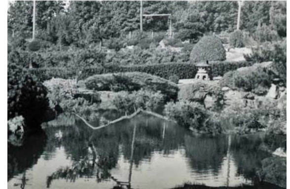
From south west corner of Japanese Garden looking north, utility poles along Renton Avenue are visible. Source: Modified version (rotated & cropped) of KGF Photo 1988a, dated 1940
