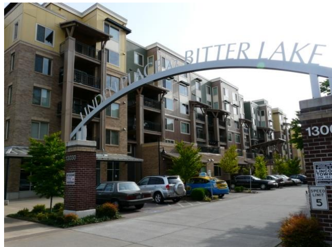
Linden Place includes 381 low-income senior and family apartments in two buildings
