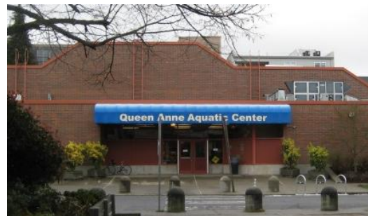
Figure 7. Queen Anne Aquatic Center, constructed 1974. Designed by Benjamin McAdoo, Jr. Photo courtesy Leanne Olson.
