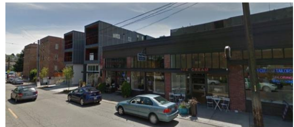
Figure 37. Block between Third Avenue W. and Fourth Avenue W. on W. Galer Street. Photo from Google Street View.
