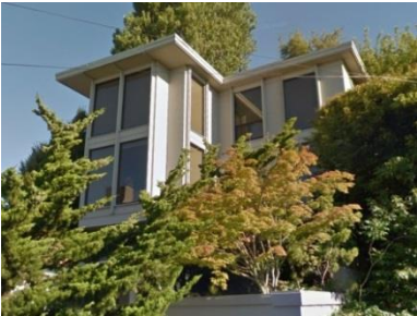
Figure 17. 18 Highland Drive, constructed 1965. Designed by Ralph Anderson (King County GIS 2015j). Photo from Google Street View.
