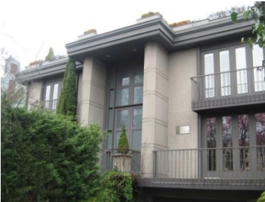
Figure 18. 610 W. Highland Drive, constructed 1967. Designed by George Hartman (King County GIS 2015k). Photo courtesy Leanne Olson.
