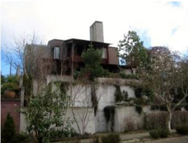
Figure 25. 1926 Seventh Avenue W., constructed 2004. Designed by Tom Kundig, Olson Kundig Architects (King County GIS 2015r). Photo courtesy Leanne Olson.
