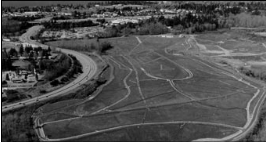
Kent Highlands Landfill – Aerial View after Closure
