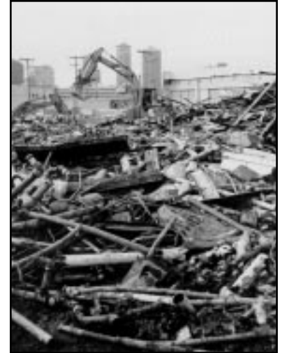
A variety of wastes are intermingled at this typical demolition site in downtown Seattle.
