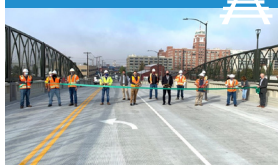
Lander St Bridge
